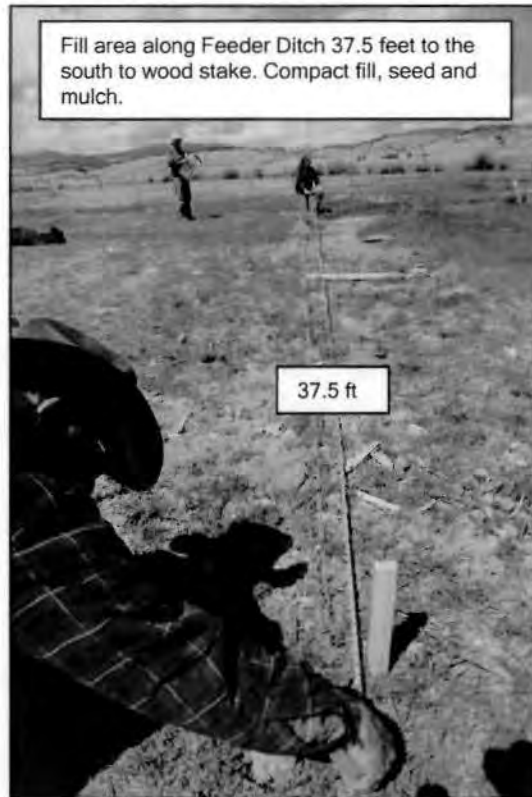
Figure F-1 Work plan for Feeder Ditch.
