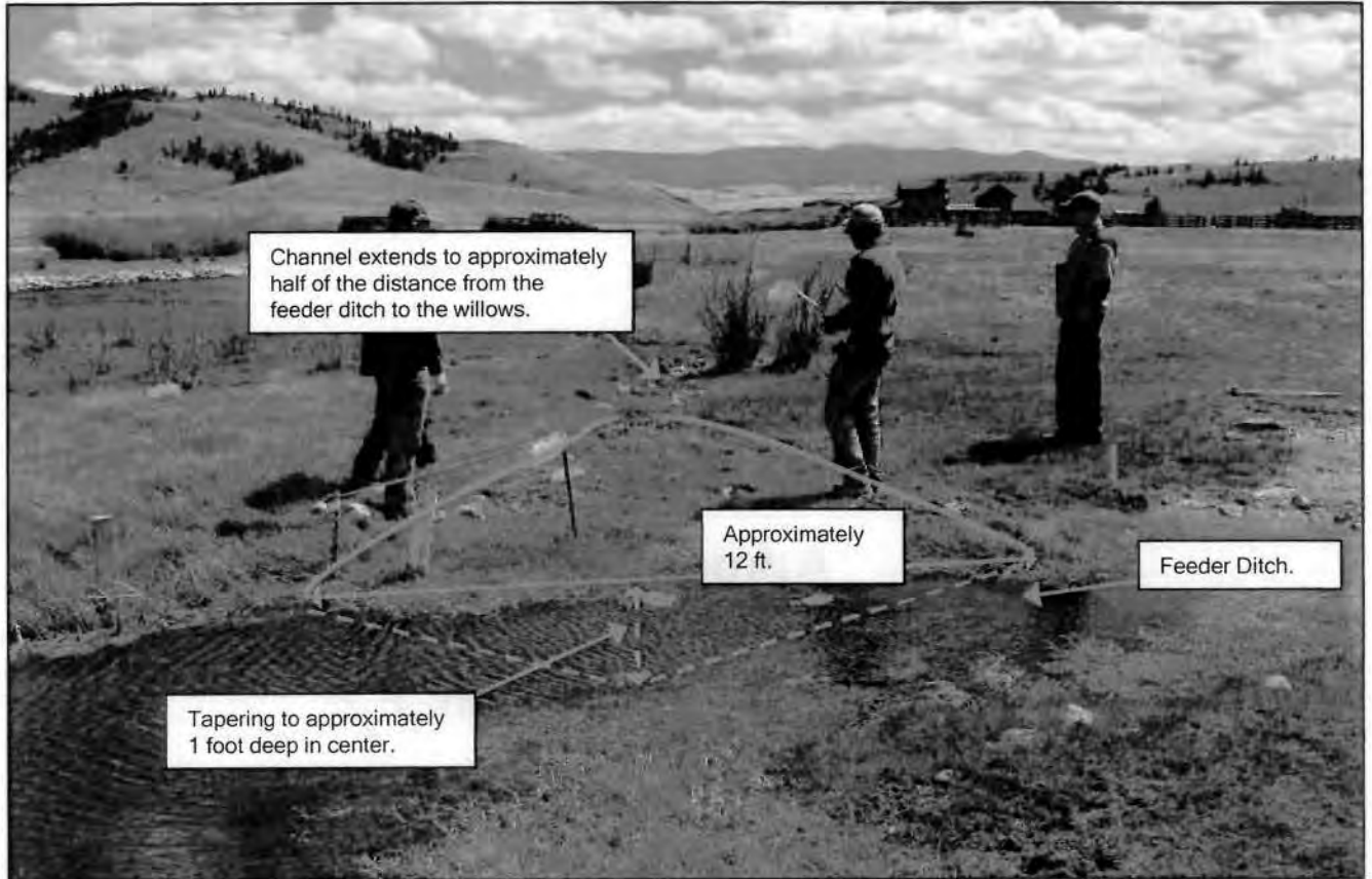
Figure F-3. Work plan for Feeder Ditch.
