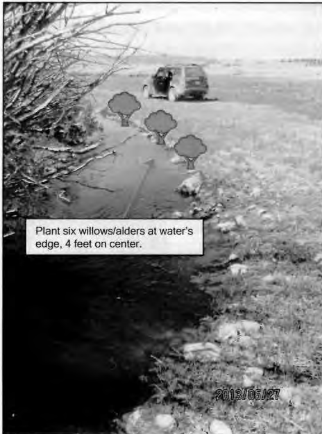
Figure E-5. bank stabilization at BS-2W. Rocks to remain since banks are wetland.
