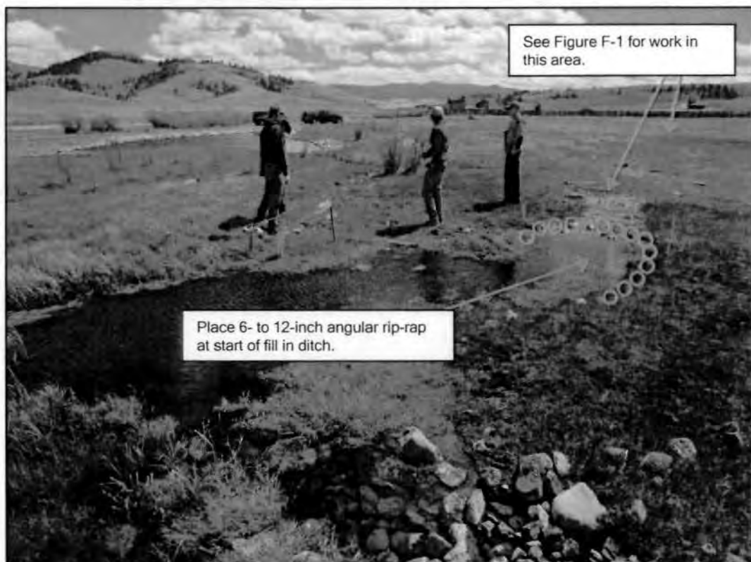
Figure F-2. Work plan for Feeder Ditch.
